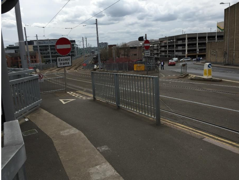
Cycle track guides cyclists to cross perpendicular to lines where road and tramline diverge, Nottingham (Adrian Lord)
